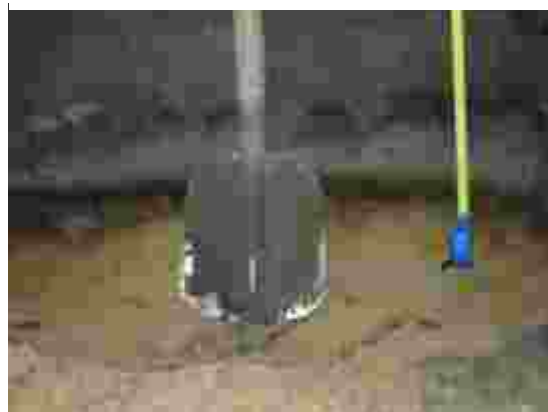
Figure III-2.2-iii.4b Example of trial pit excavated with shovel
